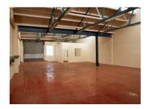
**The Triumph Trading Estate** Units have all been created by sub division of a larger building. Partition walls are formed by concrete blocks to the roof line. The roof structure is of 4 pitched bays with a mixture of traditional sheets and roof lights. A new roof has been laid over the original, providing enhanced insulation, and additional gutter capacity. Floors are concrete with a paint finish.
